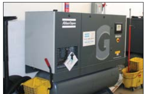
An Atlas Copco rotary screw air compressor.
