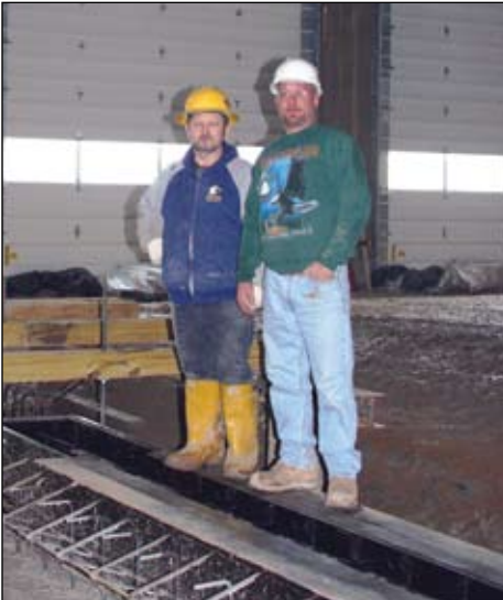
(L-R) Certified Lift Installers Joe Myszka and Daryl Lino, both of Standard Industrial, stand on a lift being installed at the City of Naperville Public Works facility.
