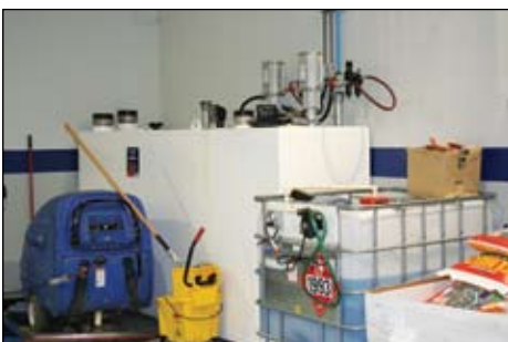
A double-walled, 800-gallon tank that can fit four products, including 5 and 10W-30 Oils.
