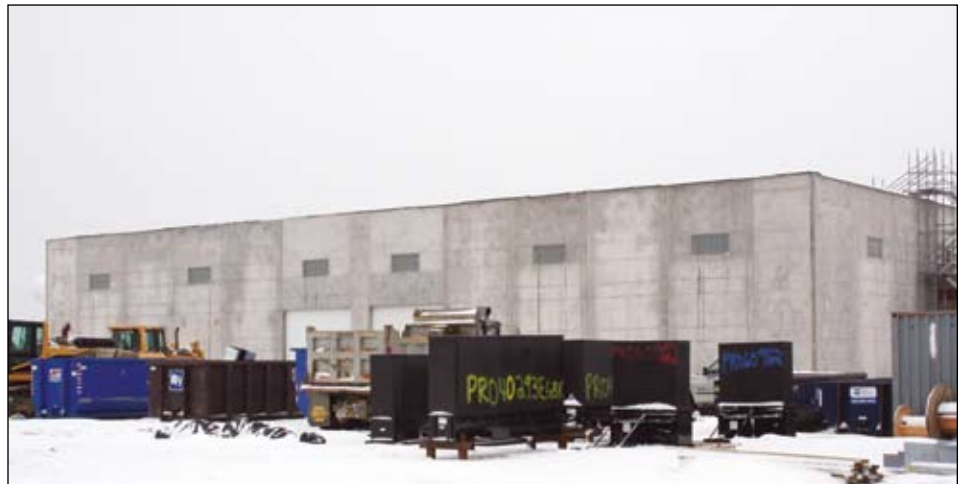
The black cassette-like objects in the middle of the photo are Rotary Mod 30 lifts before they are installed underground. These lifts have self-contained hydraulics which means there is no piping in the floor that can rust away.
