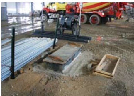
Top and Middle: Rotary Mod 30 lifts at various points of completion at the City of Naperville Public Works building. Bottom: The exterior of the 213,000 square foot facility.
